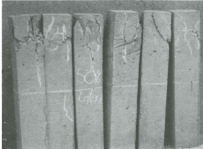
FIGURE 7: Failure Patterns of 50% Laterised Concrete with Varying Percentages of Bamboo
