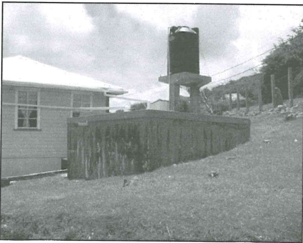
FIGURE 2: A Typical Cistern found in Carriacou, Partly Above and Below Ground
