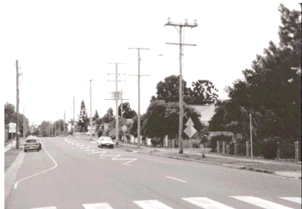
Figure 4. Zigzag markings used for warning Source: Abstracted from Queensland (2002)
