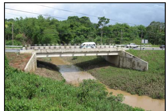
Figure 9. Replacement: 25m Beam-and-Slab
