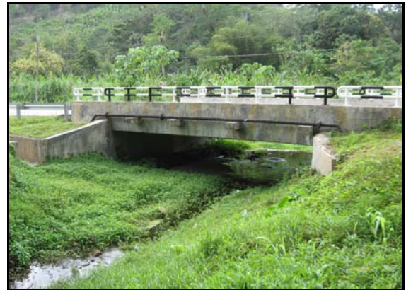
Figure 5. Replacement : 9m Box
