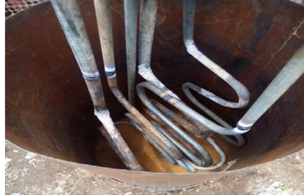
Figure 2. Combustion Chamber at Early Stage of Fabrication with Coiling of Tubes
