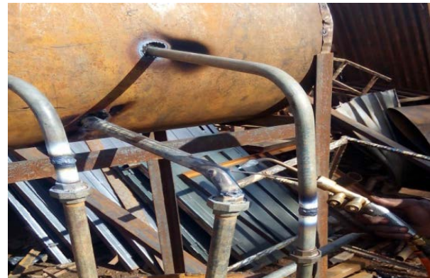
Figure 3. Steam Drum at Early Stage of Fabrication (Gas Welding)
