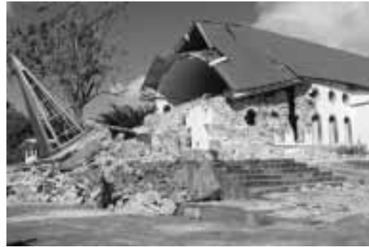
Plate 1: Damage to the St. John's R.C. Church in Portsmouth.
