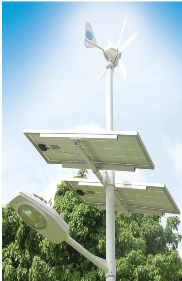
A Wind/Photovoltaic Hybrid System at the St. Augustine Campus This system not only powers a security light, but provides the added benefit of a plug and USB charging unit where persons can charge their computers and cell phones while on Campus.
