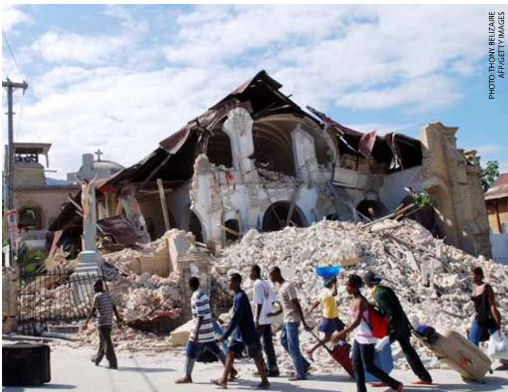
People walk by the collapsed Sacre Coeur Church in Port-au-Prince.
