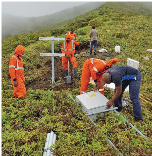
Volunteers and local community members support the team from UWI-SRC during the installation of seismic stations at the summit of the volcano. PHOTO: ST VINCENT AND THE GRENADINES NATIONAL EMERGENCY MANAGEMENT ORGANISATION
